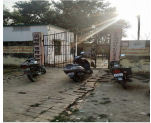
Polling Station Front View
