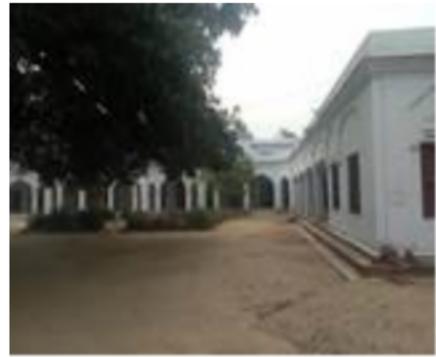
Polling Station Front View
