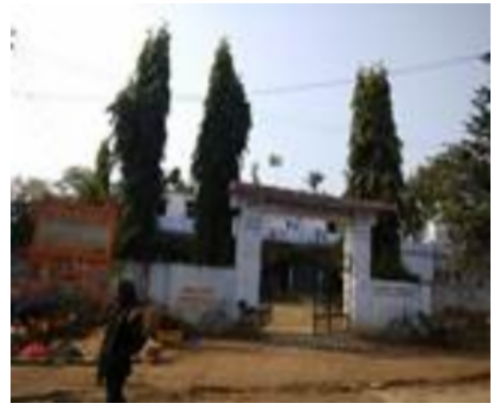
Polling Station Front View
