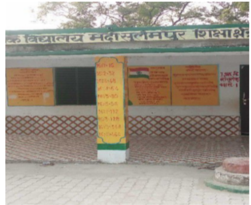
Polling Station Front View
