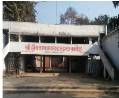
Polling Station Front View
