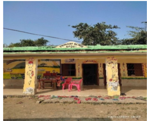
Polling Station Front View
