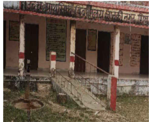
Polling Station Front View
