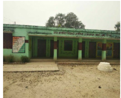
Polling Station Front View
