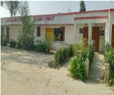
Polling Station Front View
