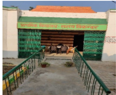
Polling Station Front View
