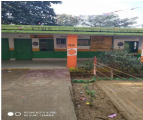
Polling Station Building Front View
