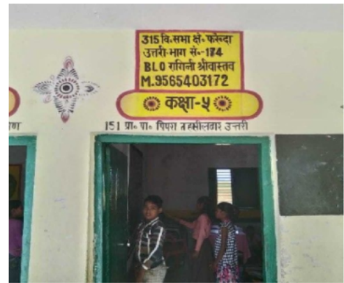
Polling Station Front View
