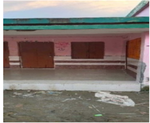
Polling Station Front View
