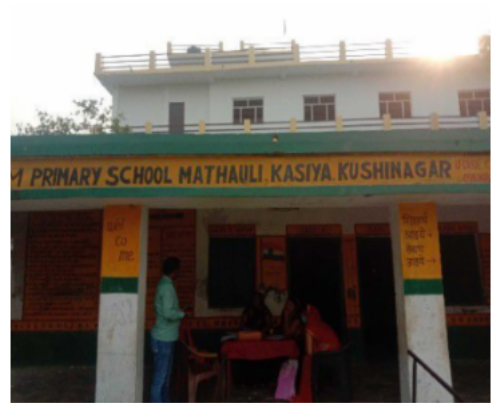
Polling Station Front View
