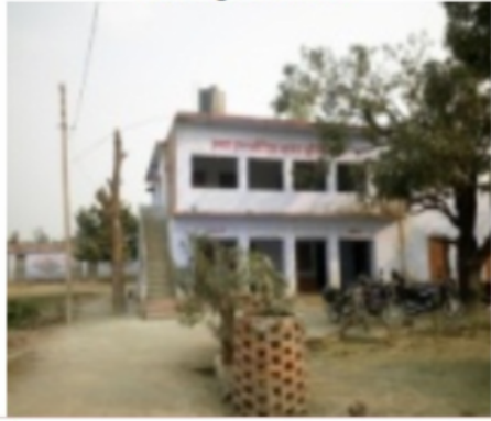
Building Front View
