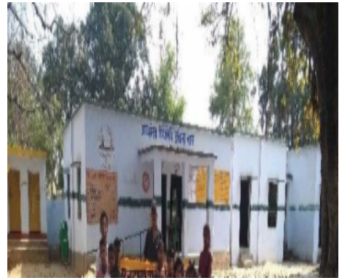
Polling Station Front View
