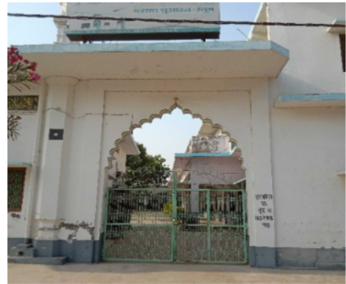
Polling Station Front View
