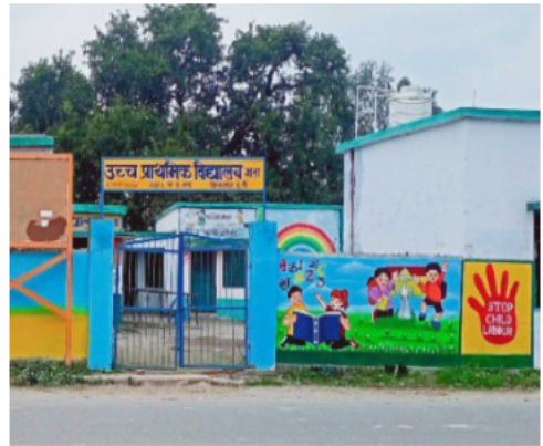
Polling Station Front View
