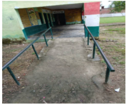
Polling Station Front View
