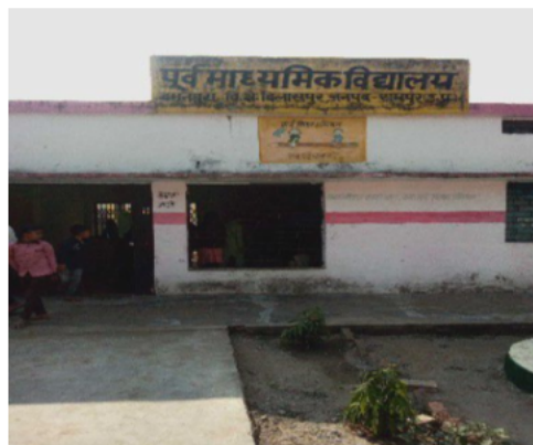
Polling Station Front View
