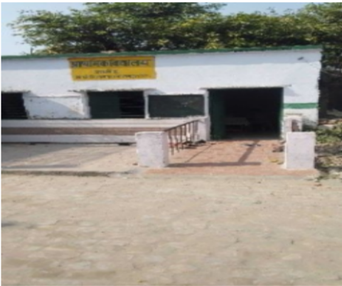
Polling Station Building Front View
