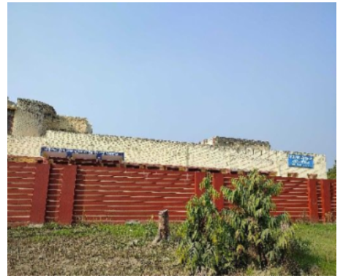
Polling Station Front View
