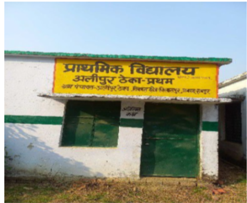
Polling Station Front View
