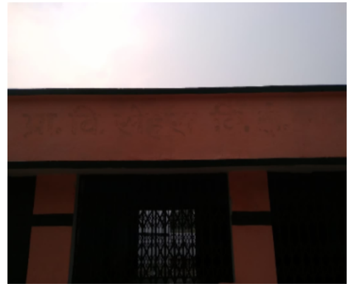
Polling Station Front View
