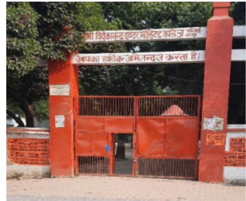
Polling Station Front View
