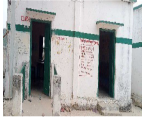
Polling Station Front View
