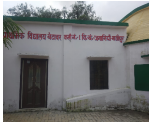
Polling Station Front View
