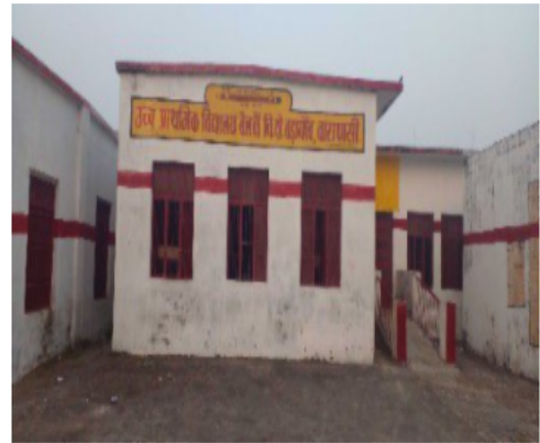
Polling Station Front View
