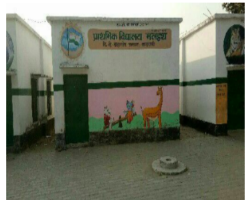
Polling Station Front View
