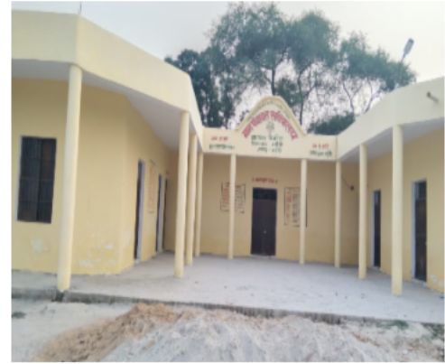
Polling Station Front View
