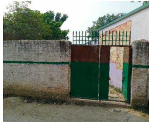
Polling Station Front View
