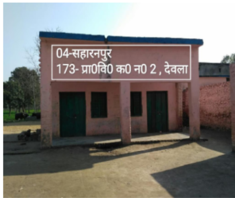
Polling Station Building Front View
