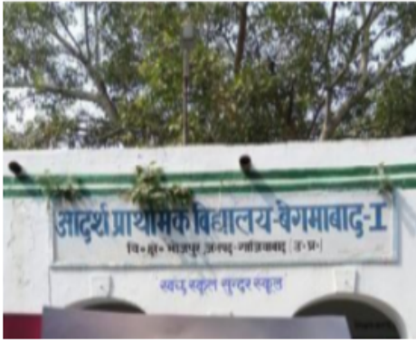
building front view
