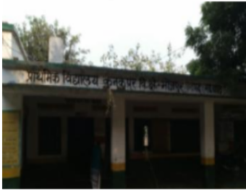
Building front view
