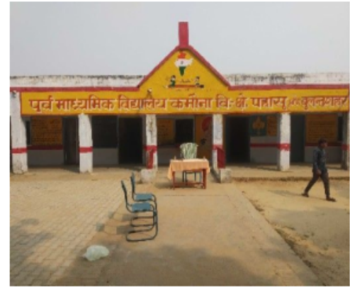
Polling Station Front View
