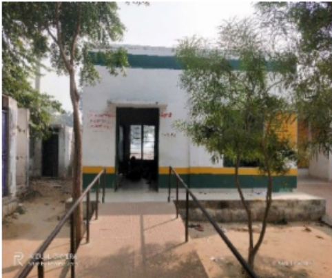
Polling Station Front View
