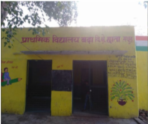
Polling Station Front View
