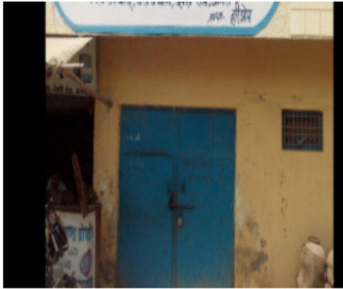
Polling Station Building Front View
