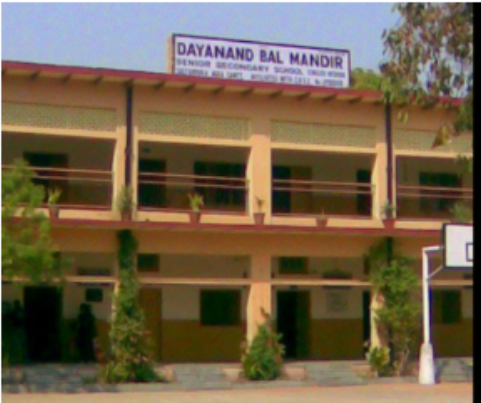
Polling Station Building Front View
