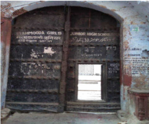
Polling Station Building Front View
