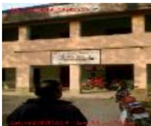
Polling Station Building Front View
