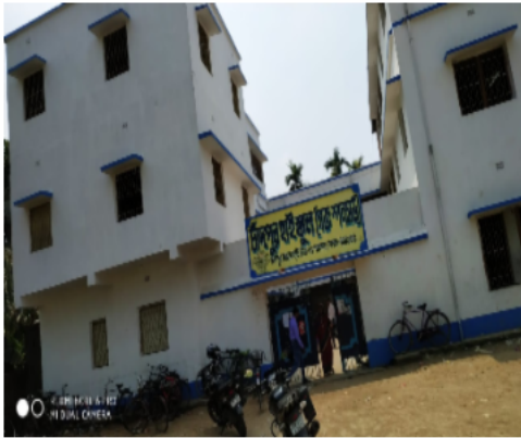
Polling Station Building Front View
