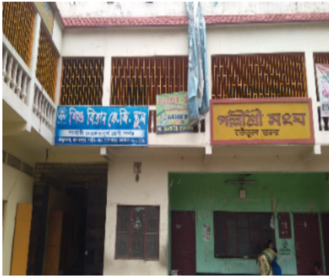
Polling Station Building Front View
