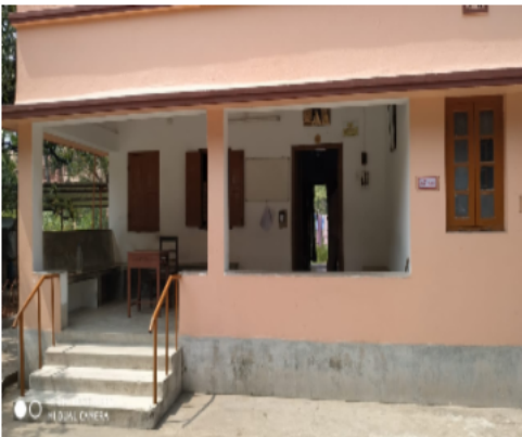
Polling Station Building Front View
