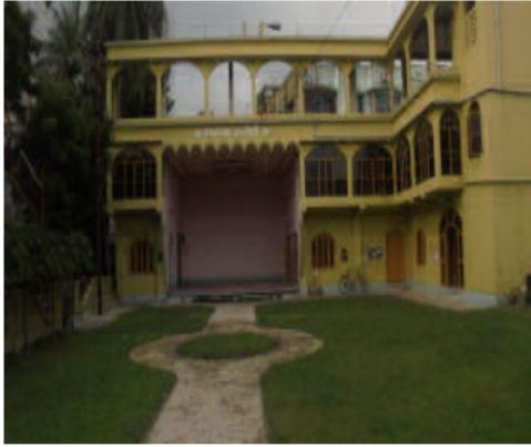
Polling Station Building Front View
