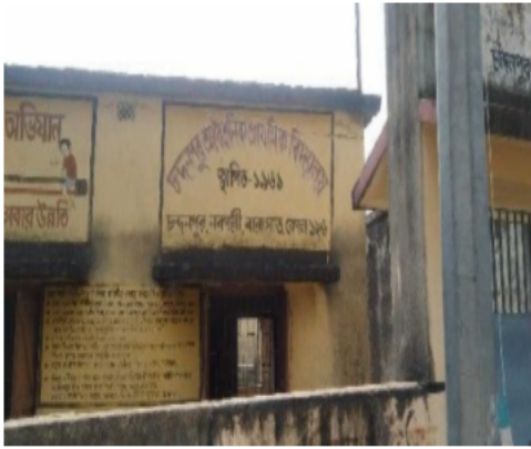
Polling Station Building Front View
