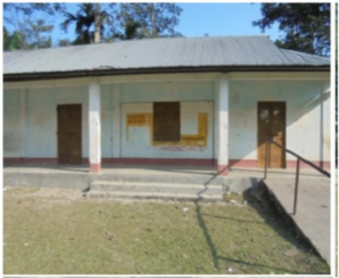
Polling Station Building Front View
