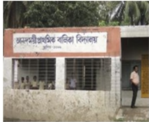
Polling Station Front View
