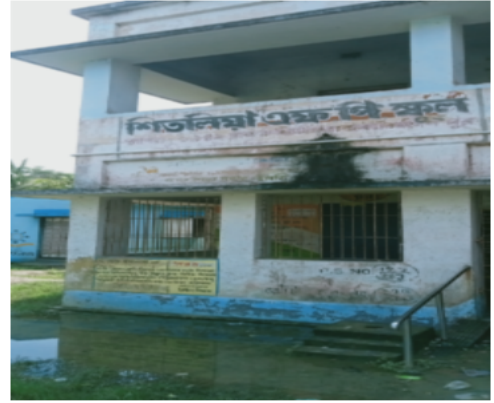
Polling Station Front View
