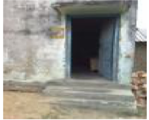
Polling Station Front View
